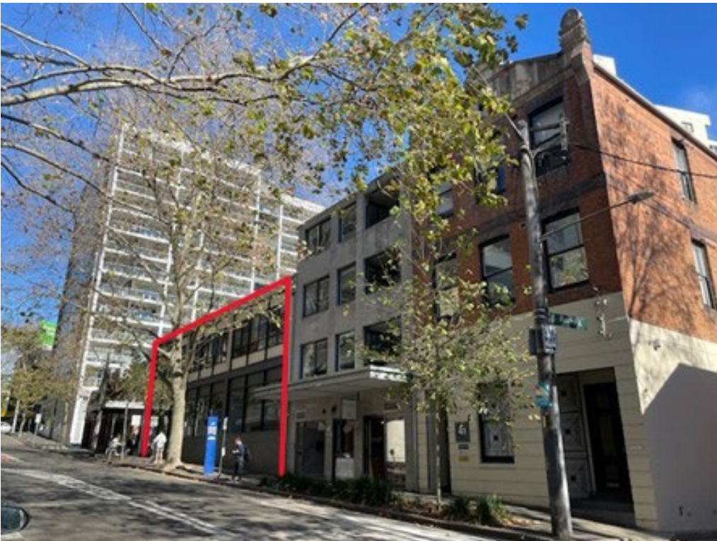
Figure 5. 47 – 51 Riley Street (outlined in red) and adjoining properties, viewed from the north-east (Riley Street frontage)
