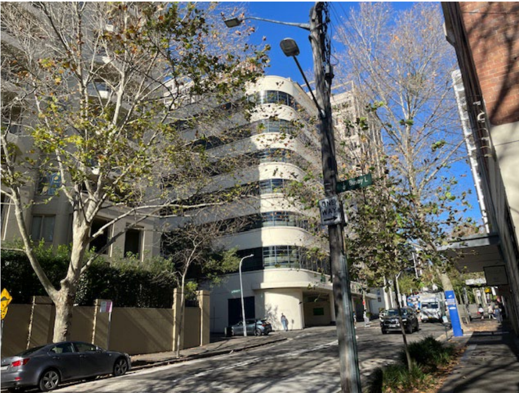
Figure 6. Properties opposite 47 – 51 Riley Street, on eastern side of Riley Street
